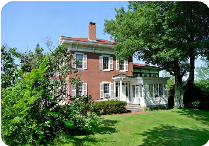
Maine Arts Commission offices, located in the historic Gage-McLean House in Augusta
